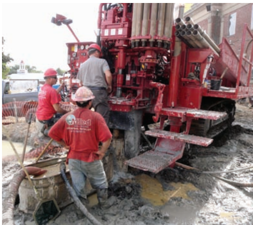
Schramm lazy susan carousel holds 15 pieces of 3 1/2-inch drill pipe
